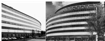
33 | Peter Behrens e Alexander Popp, Tabakfabrik Linz, 1932-33. Erich Mendelsohn, Kahfhaus Schocken, Chemnitz, 1926-1928 (Foto: Wolf Leeb).
