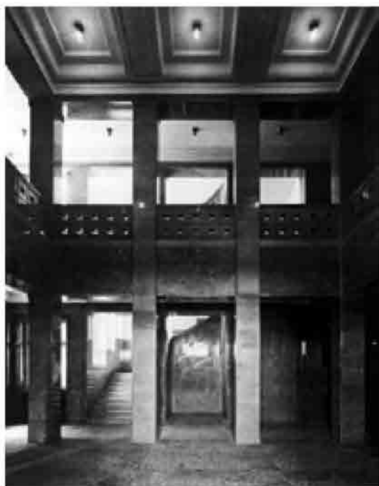
Behrens, Düsseldorf, Mannesmann Administration Building, 1910-12, Entrance hall.
