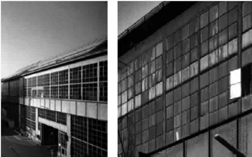
Behrens [with Karl Bernhard], Berlin, AEG Turbine Factory, west elevation, 1908-09.
