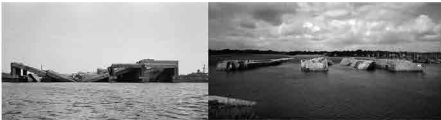
The submarine bunker Fink II immediately after the war, destroyed by the British occupying forces; the ruins of the bunker today.
